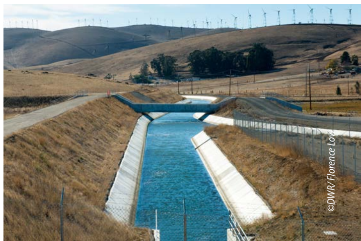
The South Bay Aqueduct consists of 8.4 miles of canals, 32.9 miles of pipelines, and 1.6 miles of tunnels. It delivers water to Alameda and Santa Clara counties.
