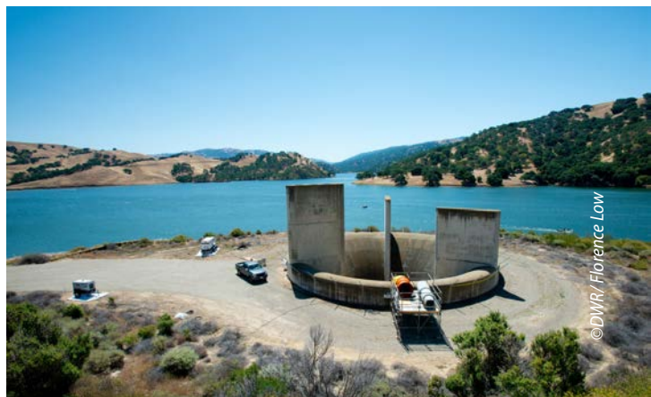
Workers inspect a tunnel at Lake Del Valle dam. Completed in 1968 as part of the State Water Project, Lake Del Valle is a storage facility for the South Bay Aqueduct
