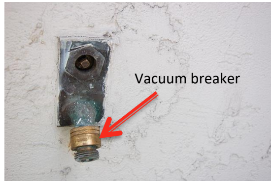
Figure 2: Vacuum Breaker
