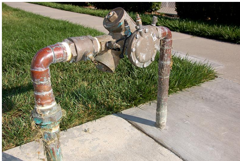
Figure 3: Reduced Pressure Backflow Prevention Device
