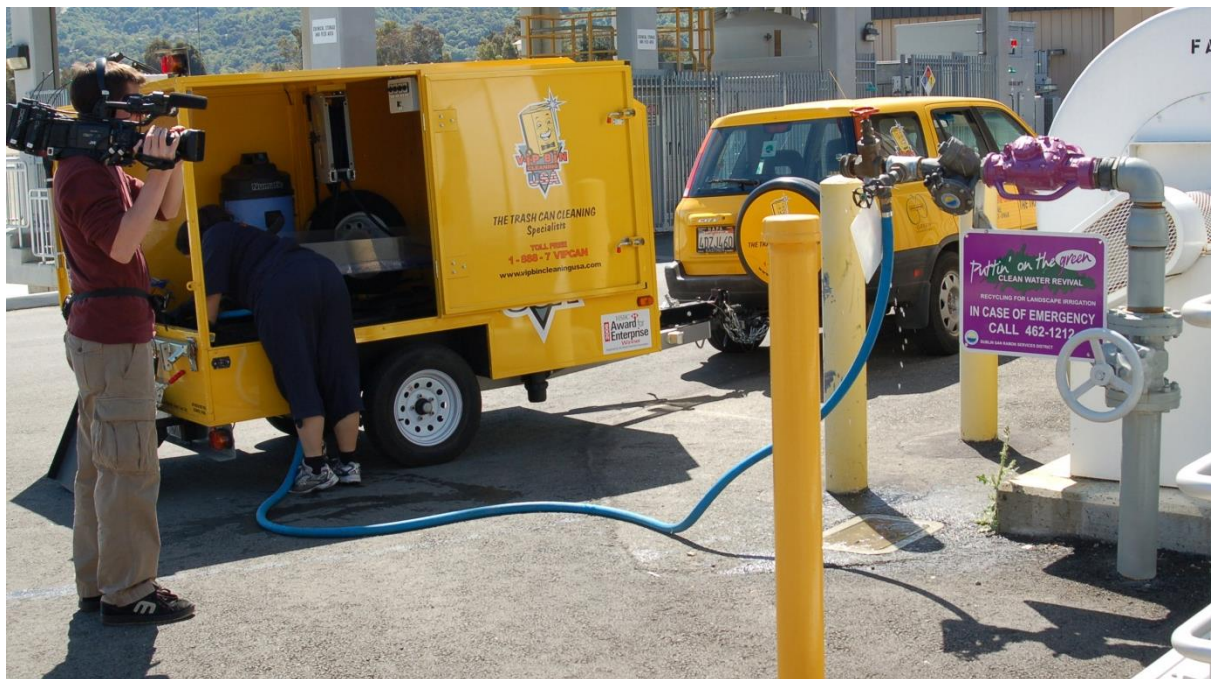
Figure 2 - A customer hooks up to the District's fill station
