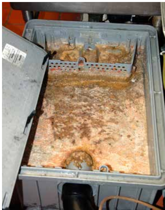
The interior of the grease trap shown at left.
