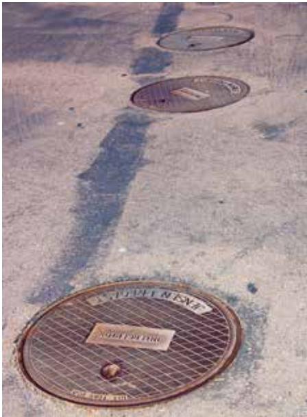
(Left) Outdoor grease interceptors: primary and secondary chambers.
