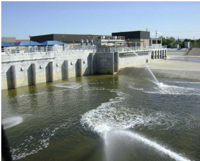
DERWA's recycled water plant is named the Jeffrey G. Hansen Water Recycling Plant for a former DSRSD director who was instrumental in bringing recycled water irrigation to the Tri-Valley.
