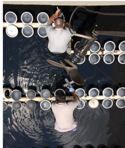
Plant operators change aeration diffusers.
