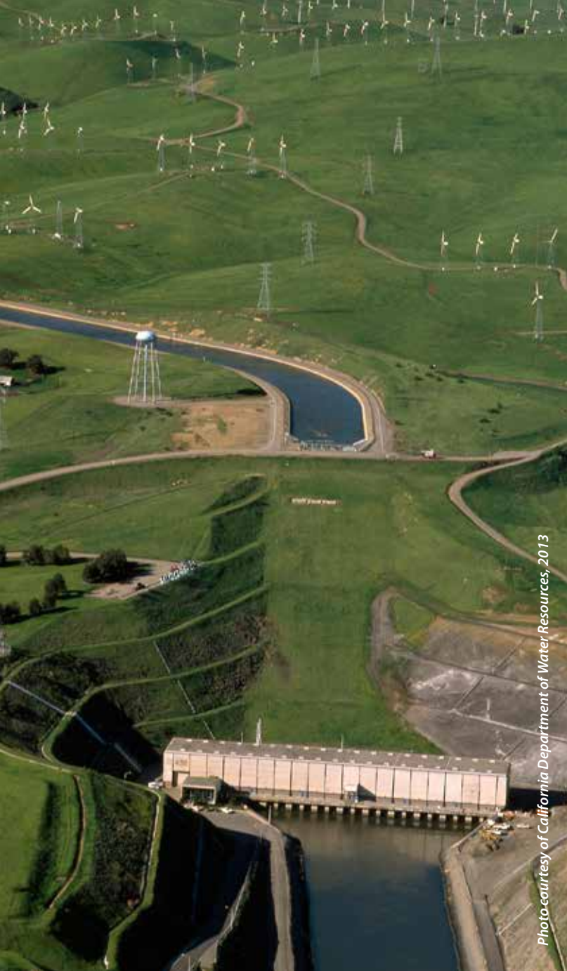
The Harvey O. Banks Pumping Plant, part of the State Water Project, is located northwest of Tracy and lifts water up into the California Aqueduct.
