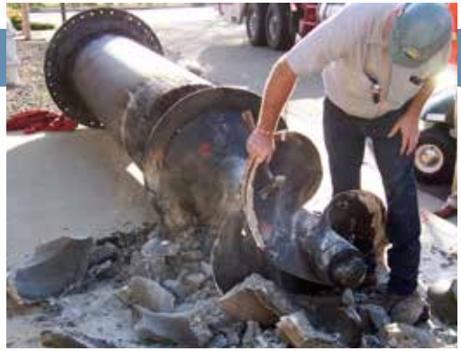
Cogen Specialist Loy Riddle (retired) chisels struvite buildup from the digester mixing blade.
