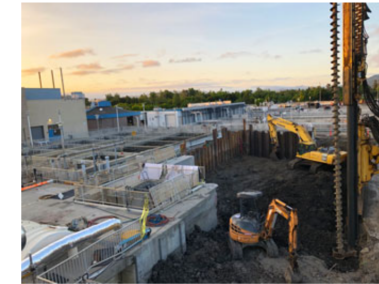
Photo: An aerial view of the demolished primary tank in May 2019.
