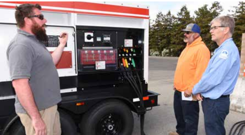
A Cummins generator instructor (left) trains Senior Mechanic Jason Miller (center) and Mechanic II Ron Freitas on how to operate the new emergency generators.
