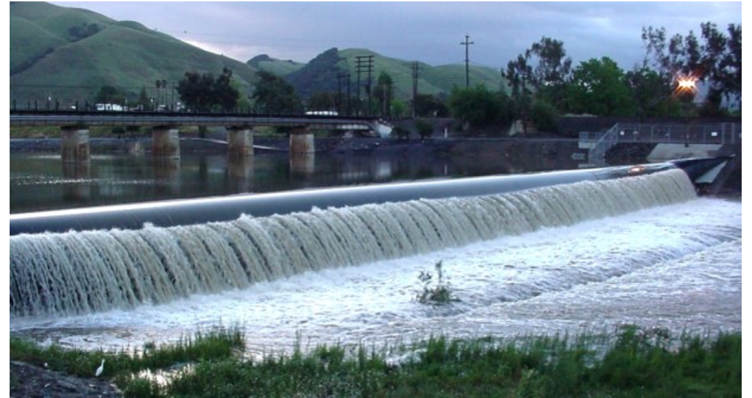
ACWD captures and diverts flow to Quarry Lakes using inflatable rubber dams on Alameda Creek.
