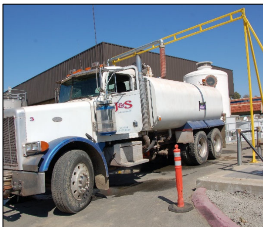
Permitted users of the commercial recycled water fill station use recycled water instead of potable water for acceptable uses.
