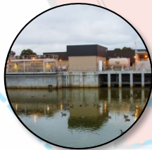
Recycled Water Treatment & Distribution (DERWA)
