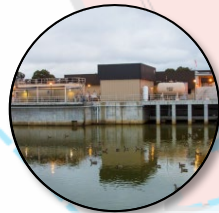
Recycled Water Treatment & Distribution (DERWA)
