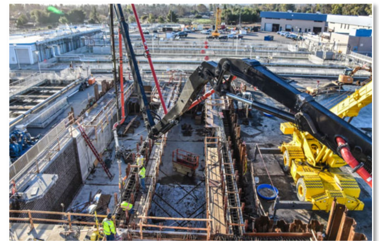
Primary Clarifier Addition
