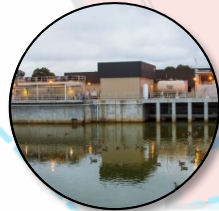
Recycled Water Treatment & Distribution (DERWA)
