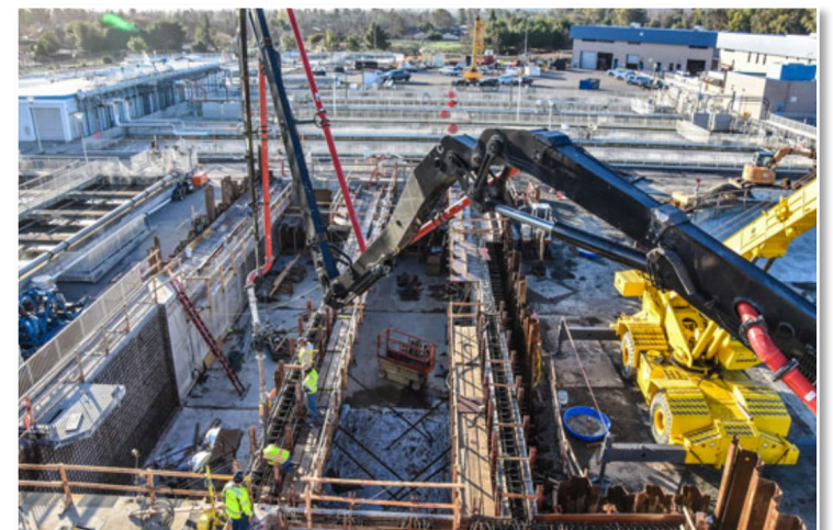
Primary Clarifier Addition
