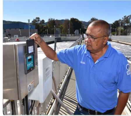
Operational improvements and optimization
