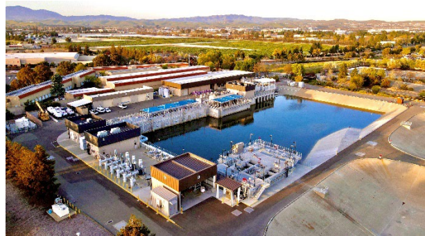
DERWA's Jeffrey G. Hansen Water Recycling Facility derives its name from a former DSRSD director who was instrumental in bringing recycled water irrigation to the Tri-Valley.
