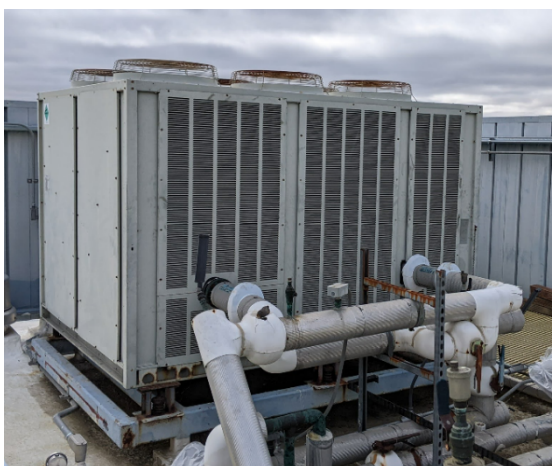
Figure 1 Air-Cooled Chiller
