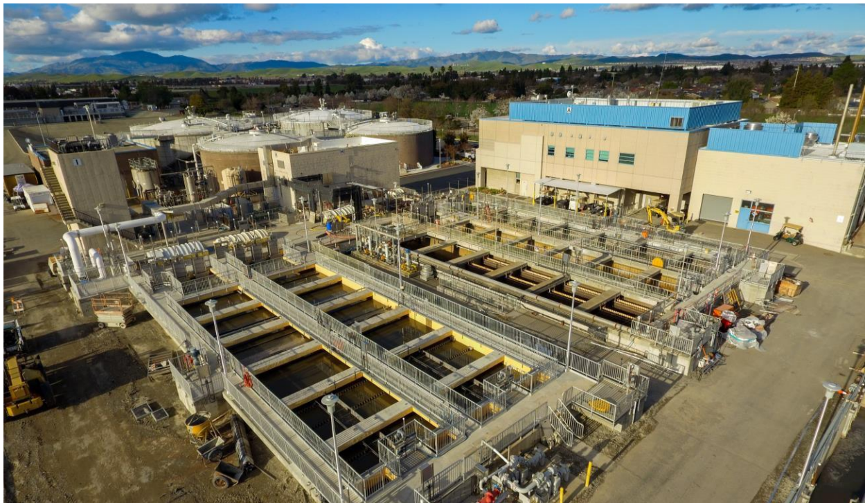
DSRSD's Regional Wastewater Treatment Facility is located in Pleasanton and treats domestic, commercial, and industrial wastewater.
