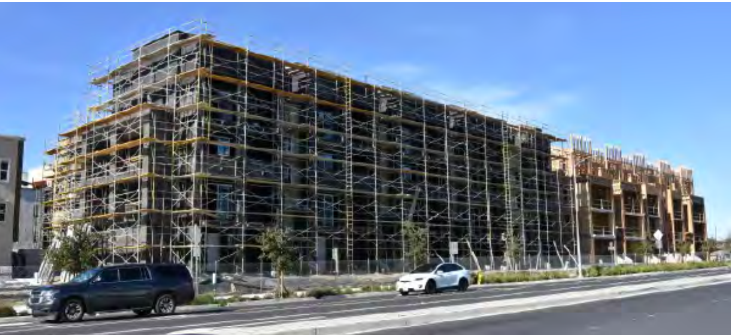
Construction continues on the former Camp Parks site.
