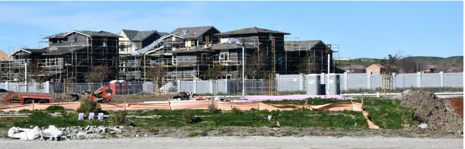
Construction continues on the Boulevard development on the former site of Parks Reserved Forces Training Area in Dublin.
