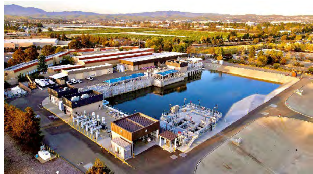
DERWA's Jeffrey G. Hansen Water Recycling Facility derives its name from a former DSRSD Board director who was instrumental in bringing recycled water irrigation to the Tri-Valley.
