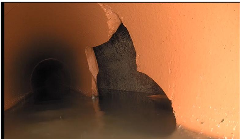
Figure 1 – Broken Pipe Void at 37 Feet
