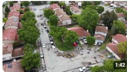
DSRSD Water Line Replacement drone flyover
